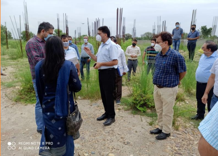
Commissioner Secretary, HED, Jenab Talat Parvez Rohella, inspecting the ongoing construction work in the college during his visit
